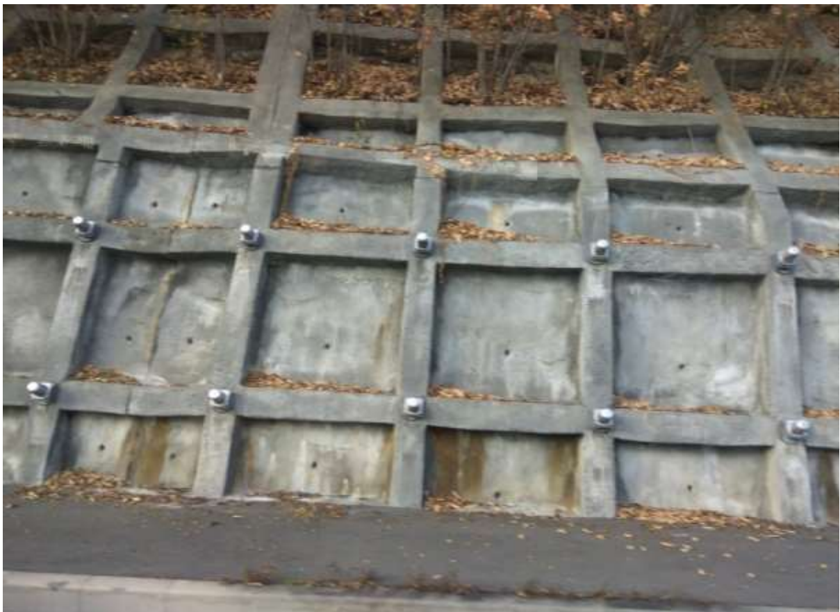
SOIL STABILIZATION WITH ANCHORING BOLT
